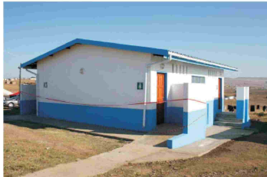
New built toilets for the St. Johns Church in Umzimkhulu
