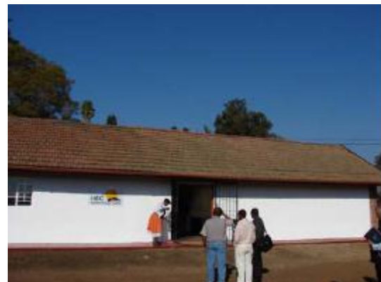
Highflats Energy Centre
