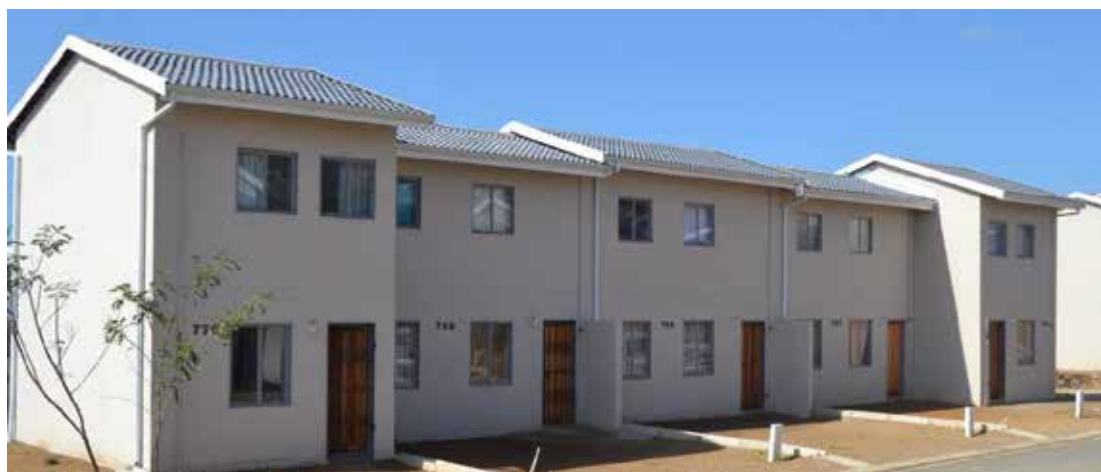
The Cornubia Phase 1B Integrated Residential Development Project (IRD). Mixed race and mixed income developments are set to be the norm.
